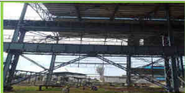
SMS B ROW COLUMN BRACING ERECTION
