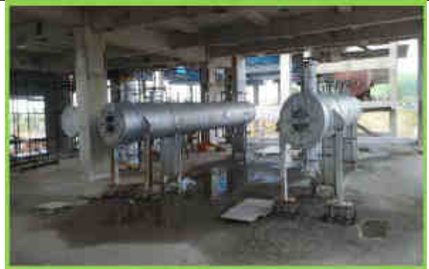
CONSTRUCTION OF HP & LP HEATER
