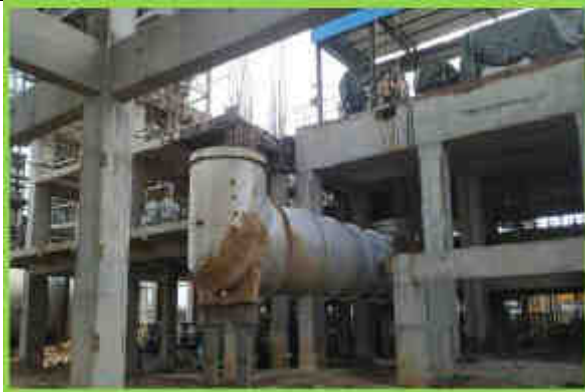
CONSTRUCTION OF DUCTING ACC
